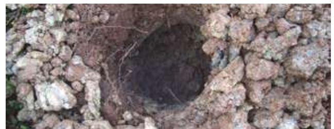
Hole digger MICROTRACTOR at work
